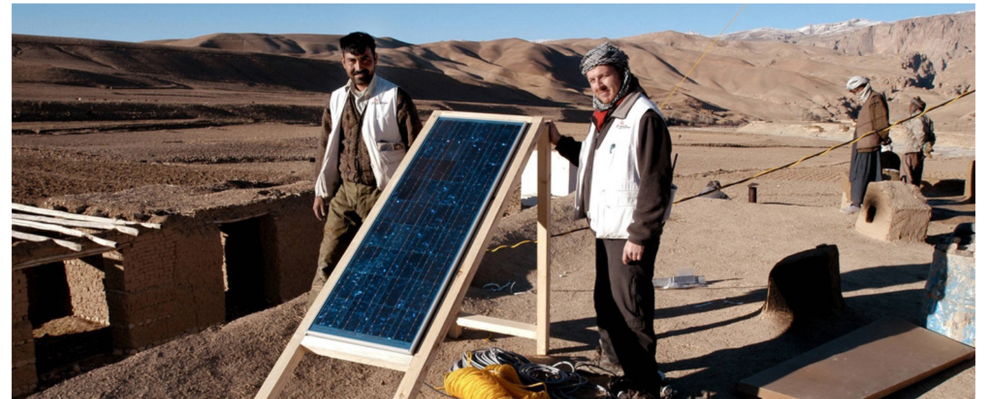
Dagah, Bamiyan Province, Afghanistan - 2003 rooftop solar panel. Jean-Marc Giboux
